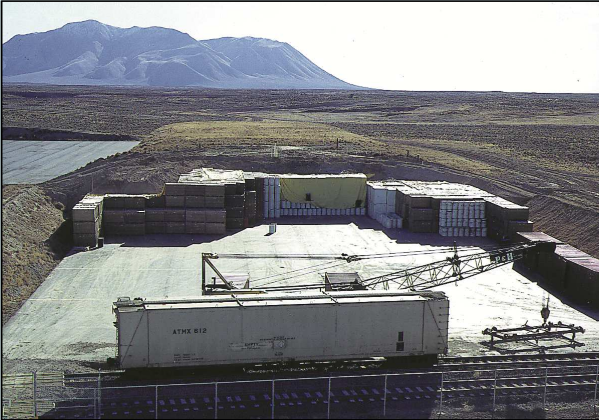
The start of above-ground transuranic waste storage in 1970s. Today, this site is covered by the Transuranic Storage Area-Retrieval Enclosure at AMWTP.
