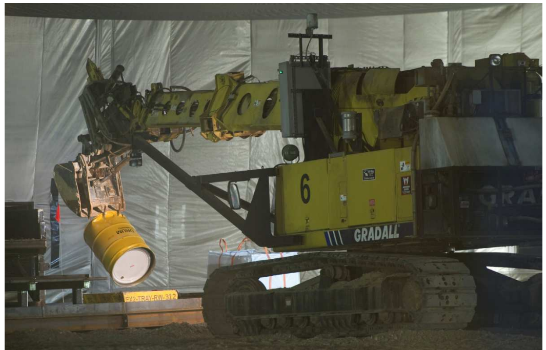
Sludge drum repackaging
