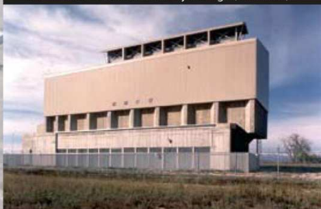
FSV-Vertical modular vault dry storage (Colorado)
