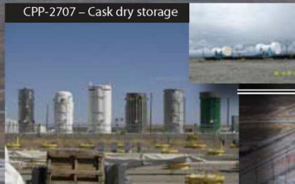
CPP-2707 – Cask dry storage
