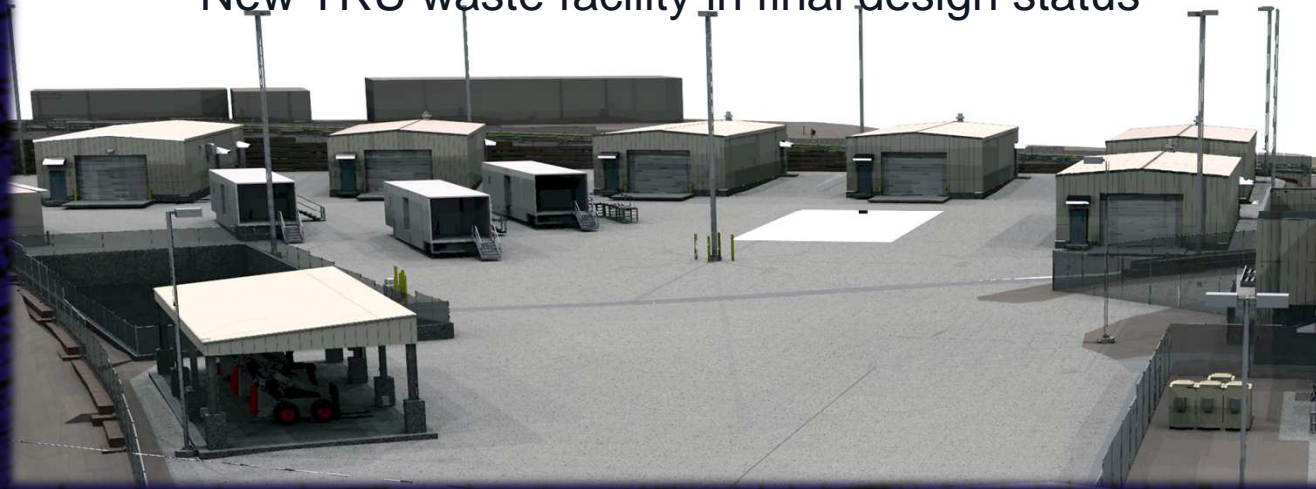
New TRU waste facility in final design status
