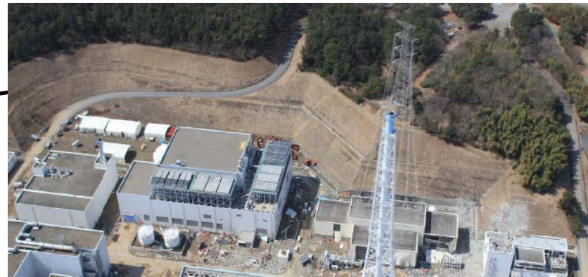
Behind buildings near Units 1-4
