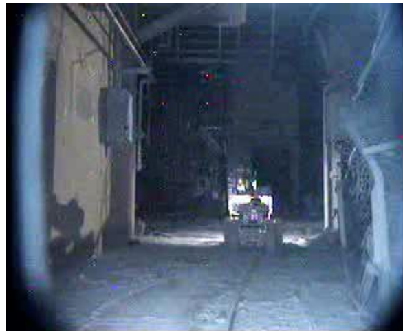
Unit-3: West Aisle 1st Floor
