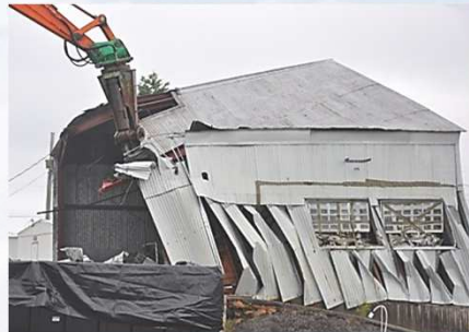
Hazardous Waste Storage Facility Demolition
