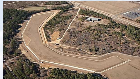
H-4 Basin Drainage Upgrades
