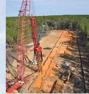
F Underground Barrier Wall
