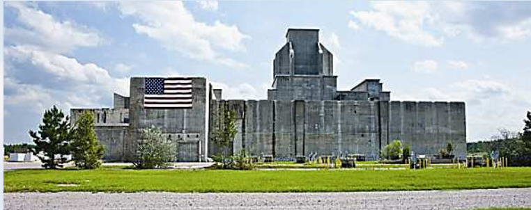
P Reactor at Completion, September 2011
