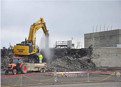
P Disassembly Basin Demolition
