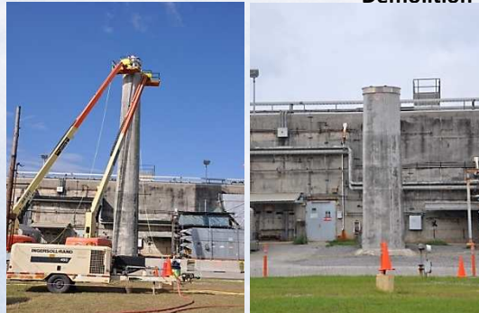
235-F Stack Reduction (During & After)
