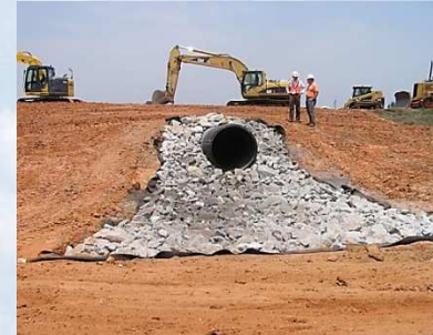
D Coal Pile Runoff Basin Drain Construction
