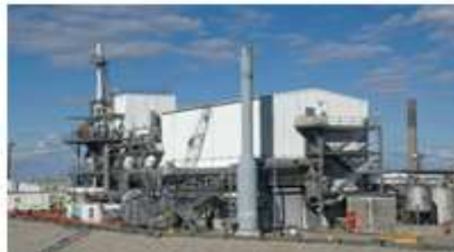
Savannah River Salt Waste Processing Facility
