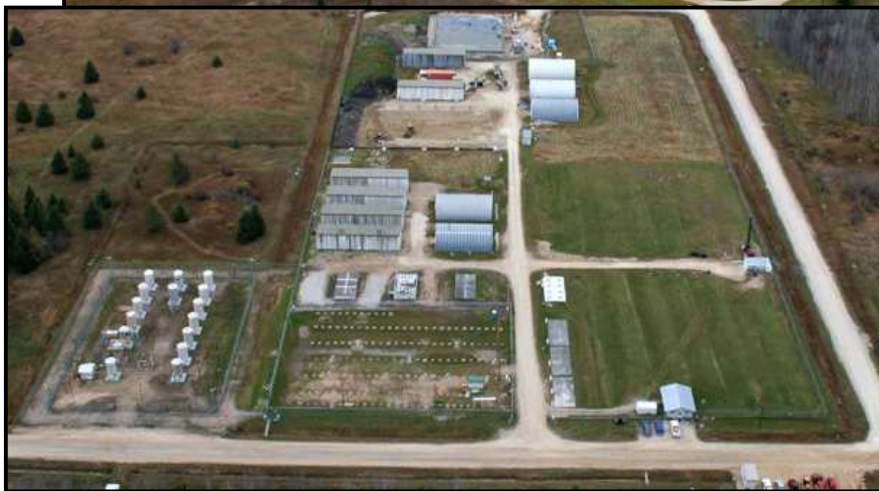
Waste Management Area from South
