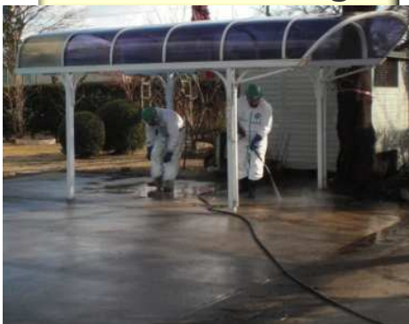
Concrete floor: High-pressure water cleaning
