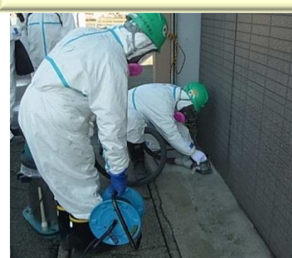
Concrete floor: Surface grinding machine
