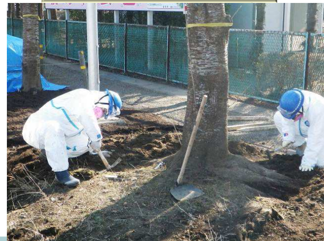
Removal of topsoil
