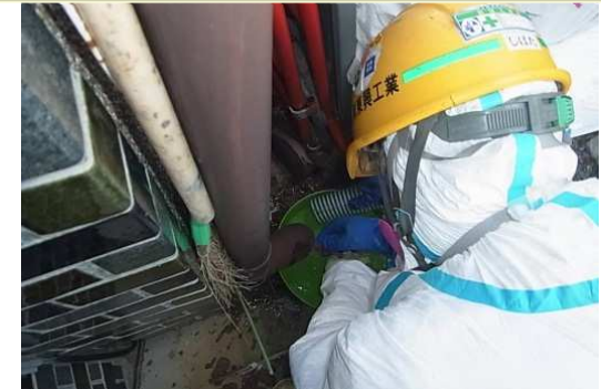
Gutter (vertical): high-pressure water cleaning
