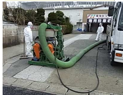
Concrete floor: Shot blast
