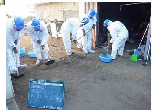
Garden: removal of topsoil
