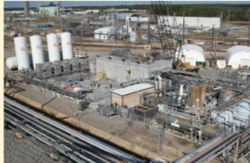
Modular Caustic Side Solvent Extraction Unit (MCU)
