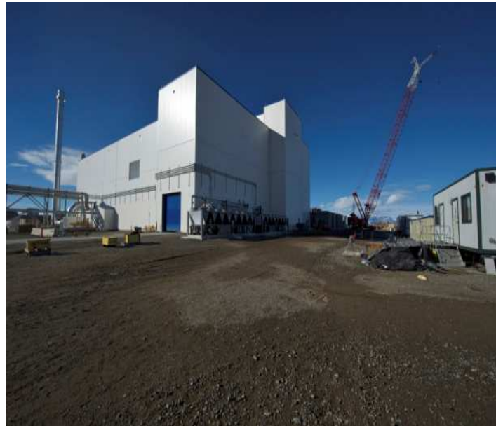
Sodium Bearing Waste Facility
