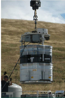
Loading drums of transuranic waste into shipping cask for shipment to WIPP
