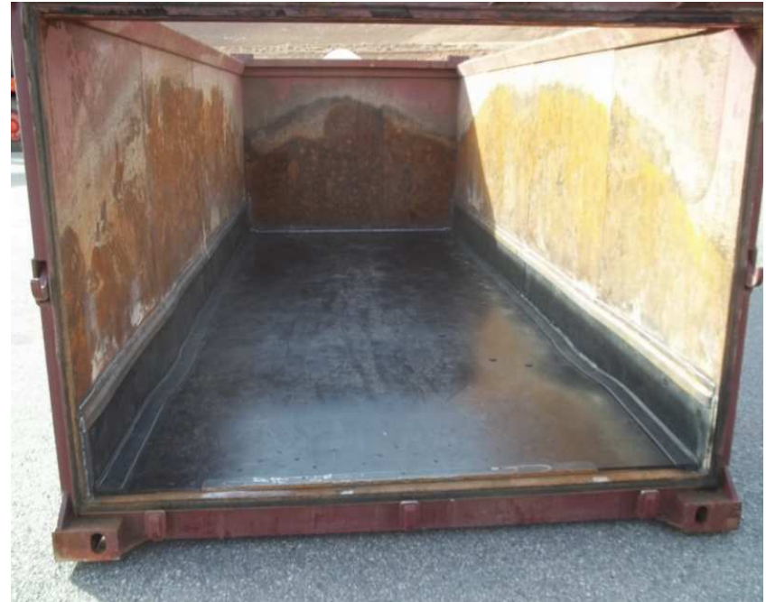
First Completed Lined Container
