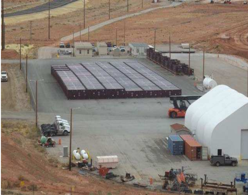
180 Staged Containers on Ground in Queue for Permanent Liner Installation
