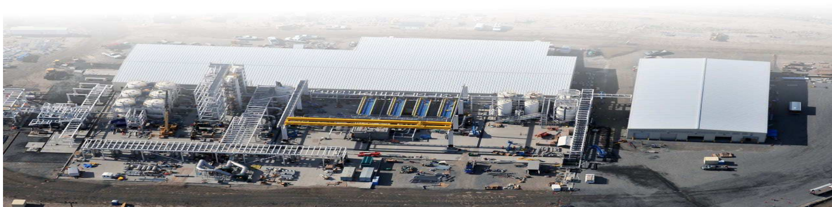
Aerial view of the 200 West pump and treat facility at Hanford.
