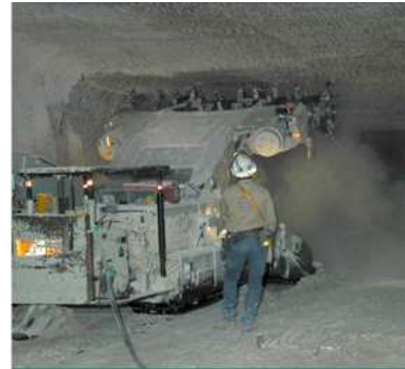
Continuous mining machine used to excavate rock salt to create underground disposal areas
