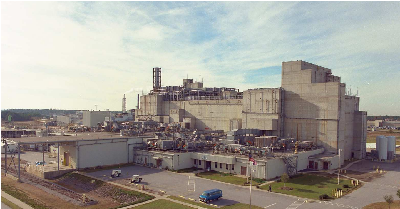
Defense Waste Processing Facility
