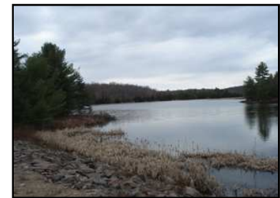
Uranium mine and mill tailings
