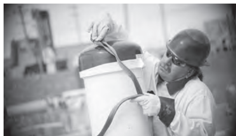
A crane and rigging worker prepares to lift equipment into position near C-104, one of three underground waste storage tanks emptied this year at Hanford.
