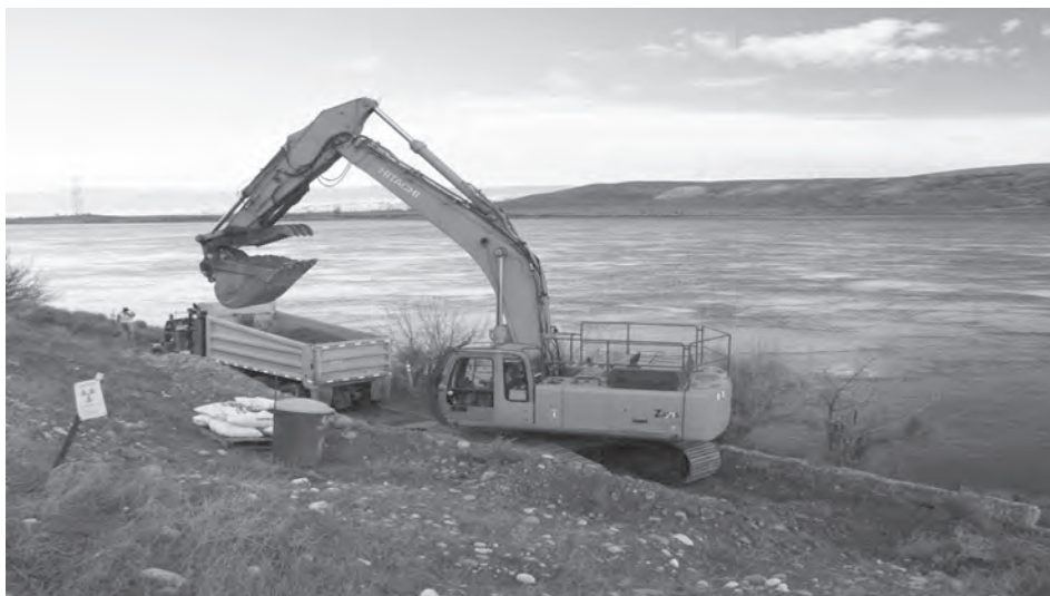
Workers excavate contaminated soil from an F Area waste site near the Columbia River.
