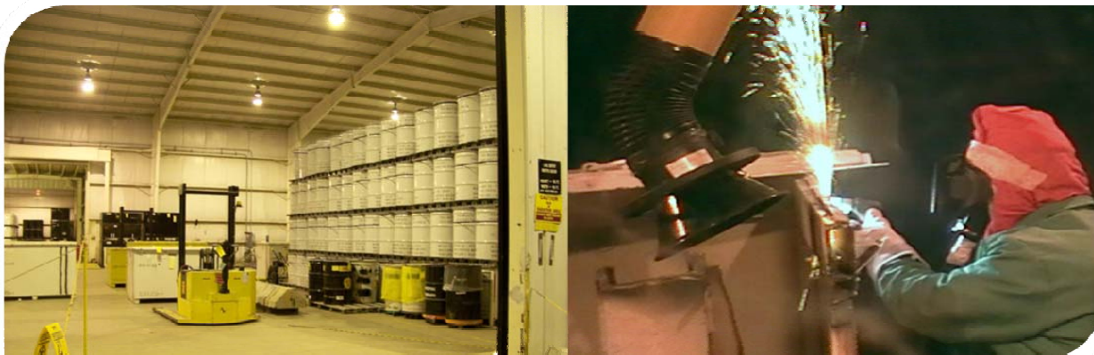
Fig. 3. RH and CH TRU waste processing (right) ramped up over the past four years. Once processed per the WIPP waste acceptance criteria, the TRU waste is placed in on-site storage for eventual disposition (left).
