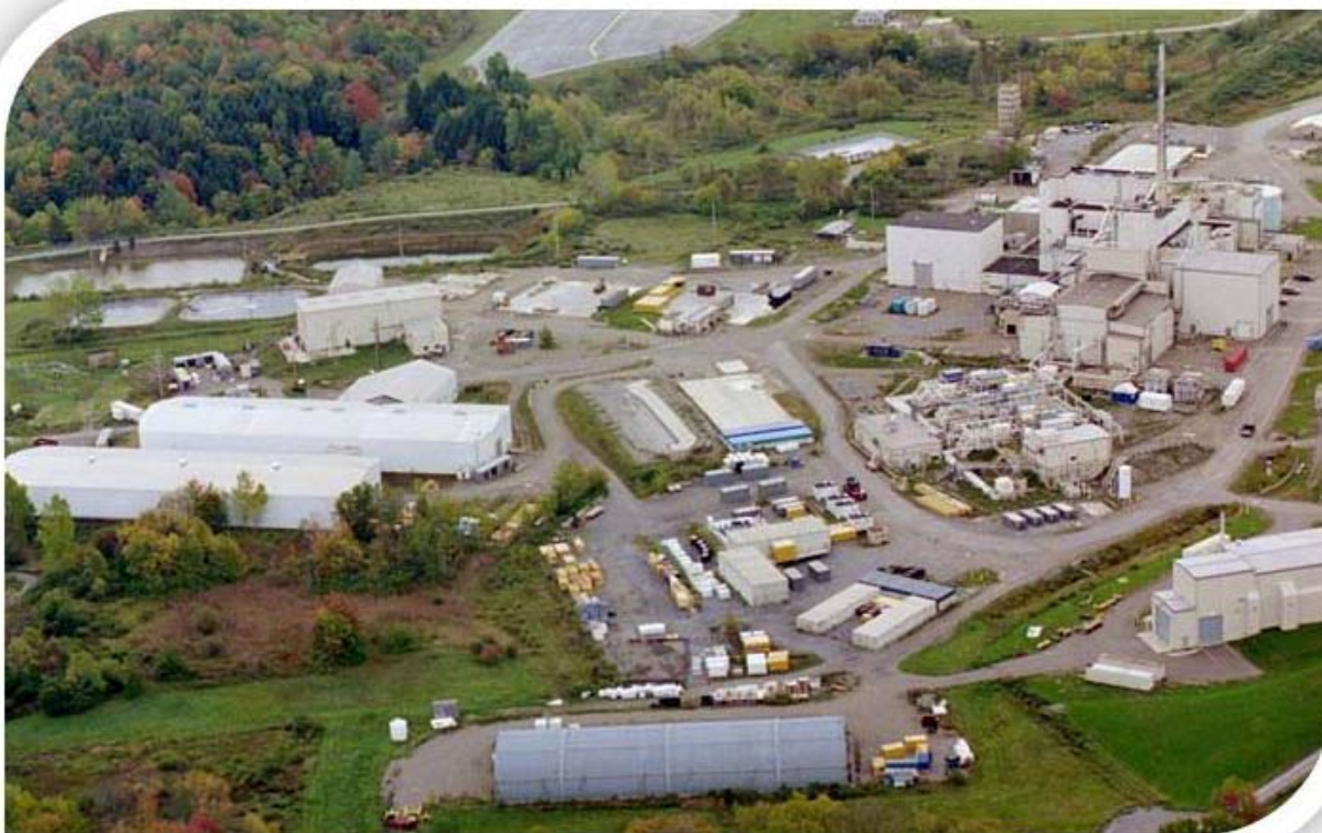
Fig. 1. At its peak, the Project had nearly 28,300 m 3 of legacy waste in storage in tent-like structures and hardstands awaiting off-site disposal.
