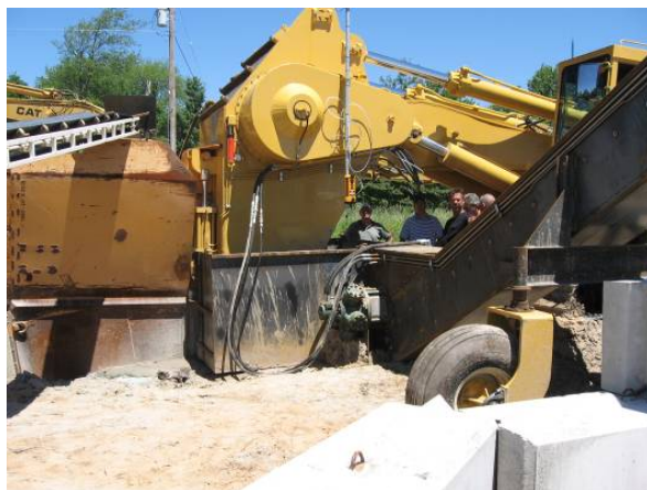
Fig.5. Testing of conveyor.
