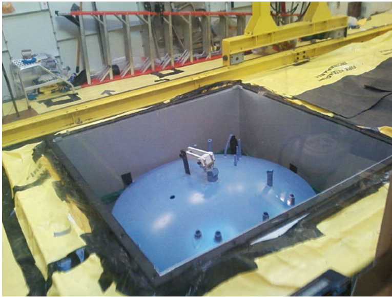
Figure 4: Tank 7D-1, the first vessel removed from XC-1, was safely removed from cell and placed in a staged waste container in the hatch opening of XC-2 in early November 2010. The top of the vessel is shown above.
