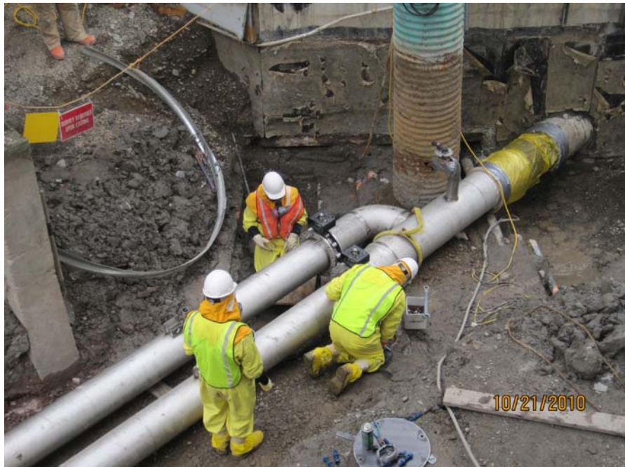
Fig. 3. Installation of new underground ventilation line.
