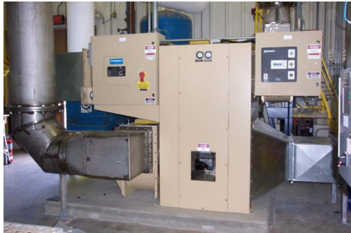
Fig. 2. Munters Rotary Dryer, Model HCD-4500.
