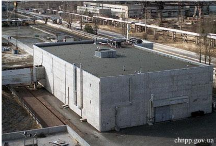
Fig. 1 .Liquid Radioactive Waste Treatment Plant (LRTP)
