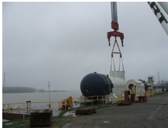
Figure 3. Transferal of steam generator from barge to over the road transport
