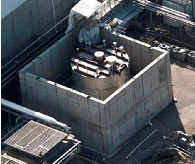
Fig 2. Waste Concentrate Hold Tank (WCHT) installed at ETP to collect low level waste.
