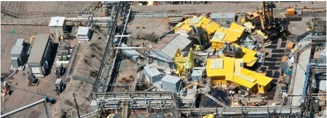
Fig 4. Tank 13 – Recovery Act funding installed pumps, upgraded ventilation, hydrogen monitoring, electrical equipment and shielding to allow bulk sludge removal from the tank.
