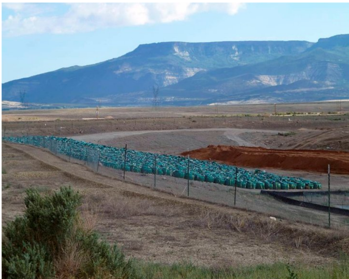
Figure 3. Bags of radioactive material ready from Highway 160 site placed in Grand Junction Disposal Cell.
