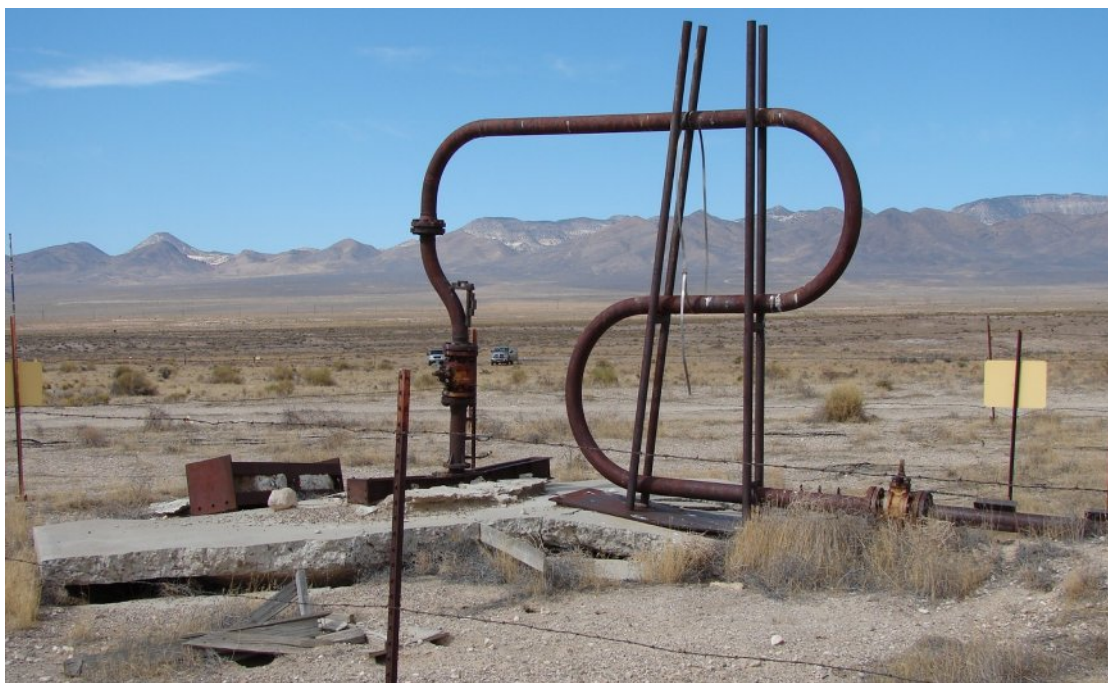
Fig 2. NNSS CAU 547 internally contaminated piping – ongoing Industrial Sites activity.
