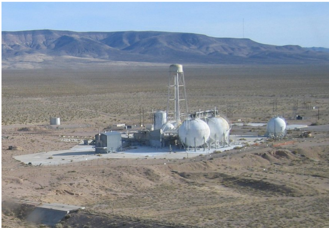
Fig 1. NNSS CAU 116 Area 25 Test Cell C Facility – remediated under Industrial Sites.
