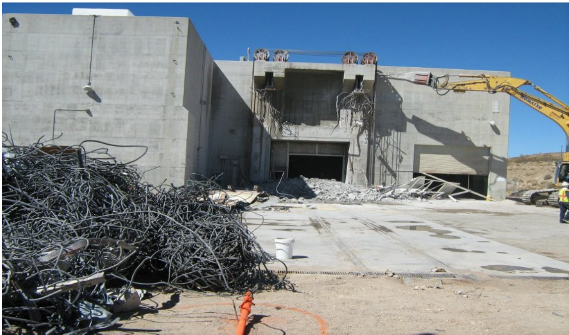
Fig 4. NNS CAU 117 Pluto Facility – undergoing Industrial Sites demolition.
