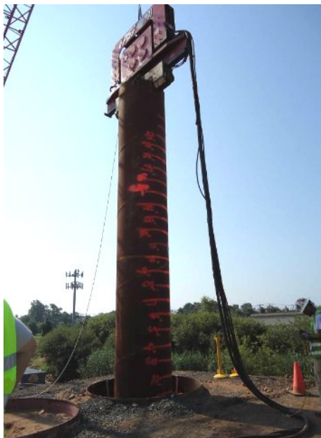
Figure 6: Over-casing with vibratory hammer
