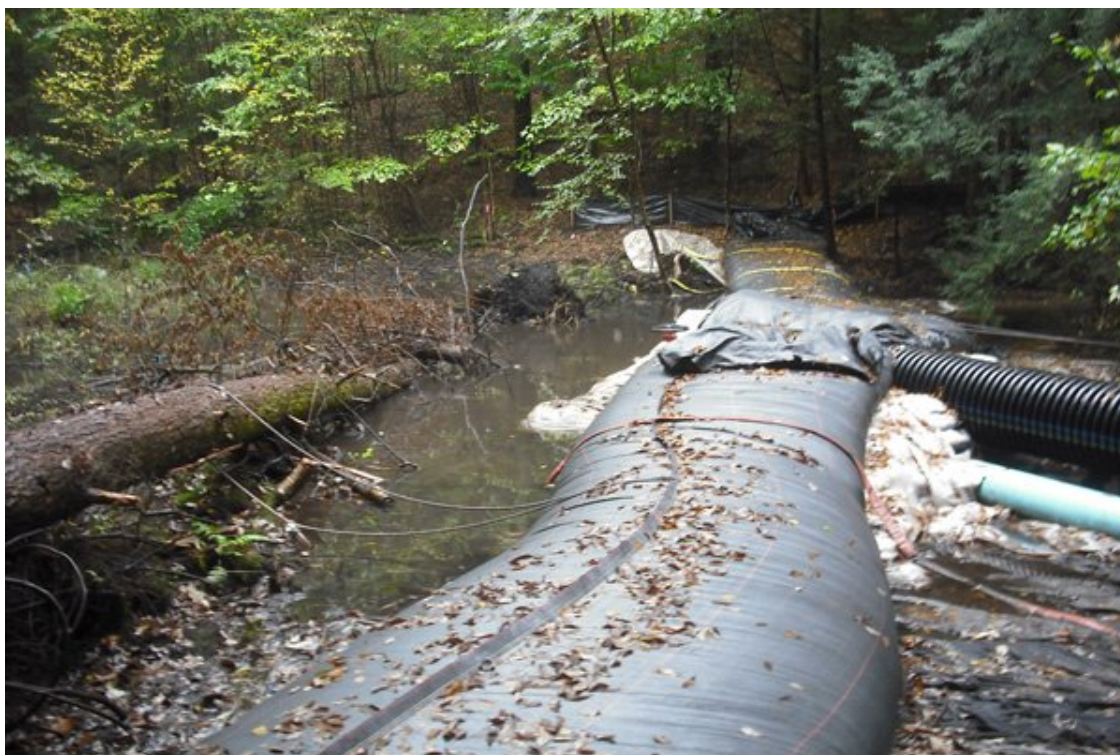
Fig 1. Water diversion using bladder berms.
