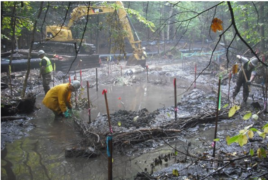
Fig 2. Excavation activities in an area of Site Brook.
