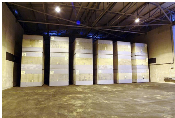
Figure 10 WAGR Waste Box Store
