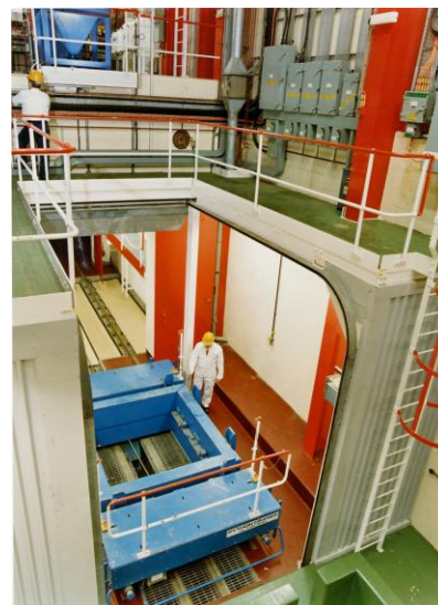
Figure 8 Waste Packaging Building – Transfer Station
