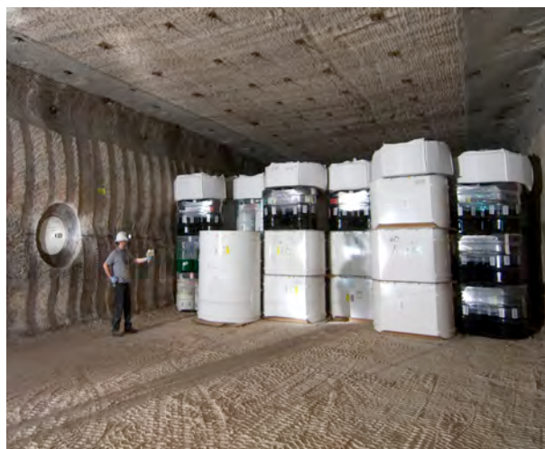
Fig. 3. Over 10,000 nuclear waste drums and standard waste boxes filling 1 of 56 rooms to be filled at WIPP over a 20-year period. Over 30 rooms have been filled as of September 2011. Note the high-activity remote handled waste (RH) plunged into boreholes in the wall to the left and plugged, while the contact handled waste (CH) fills the bulk of the room. The technician shown is receiving about a tenth of the radiation dose that we receive at the Earth's surface, ironic since he is standing in front of the nuclear waste.
