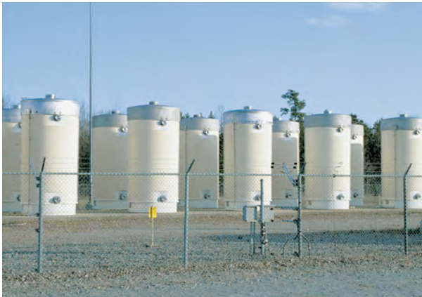
Fig. 1. (above) Wet storage of spent nuclear fuel in pools of water. When spent fuel is removed from the reactor it requires about five years in water to cool off and allow the short-lived radionuclides to decay away. It can then transferred to dry cask storage (below) until needed, e.g., burned in Generation IV or V fast reactors in the near-future.
