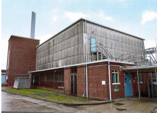
Fig 1: The Facility showing the Ground Floor Access
