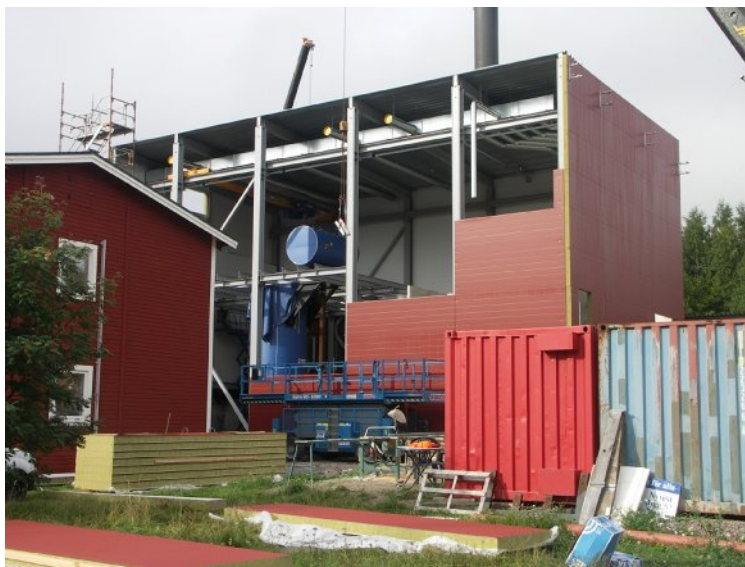
Figure 4 Pyrolysis plant partly built
