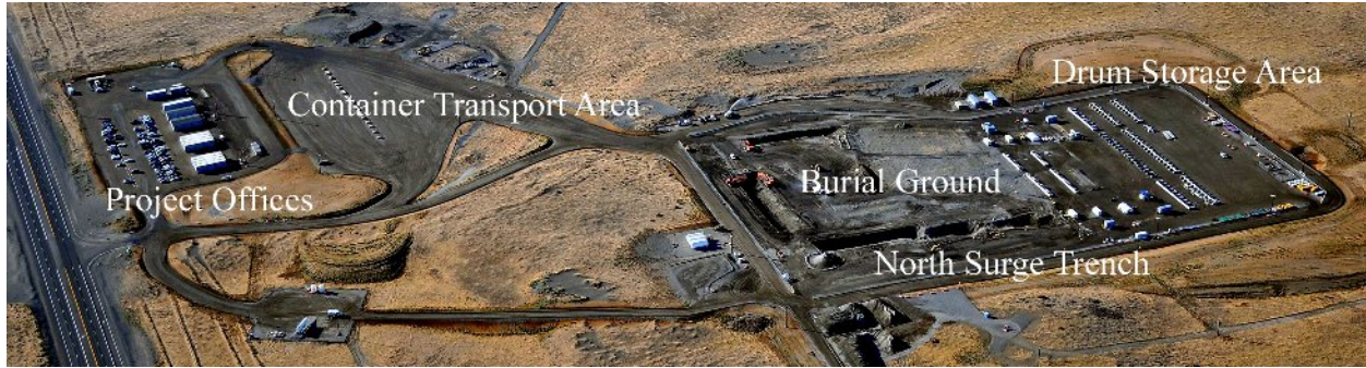
Fig 1. Location of the 618-10 Burial Ground and site facilities.
