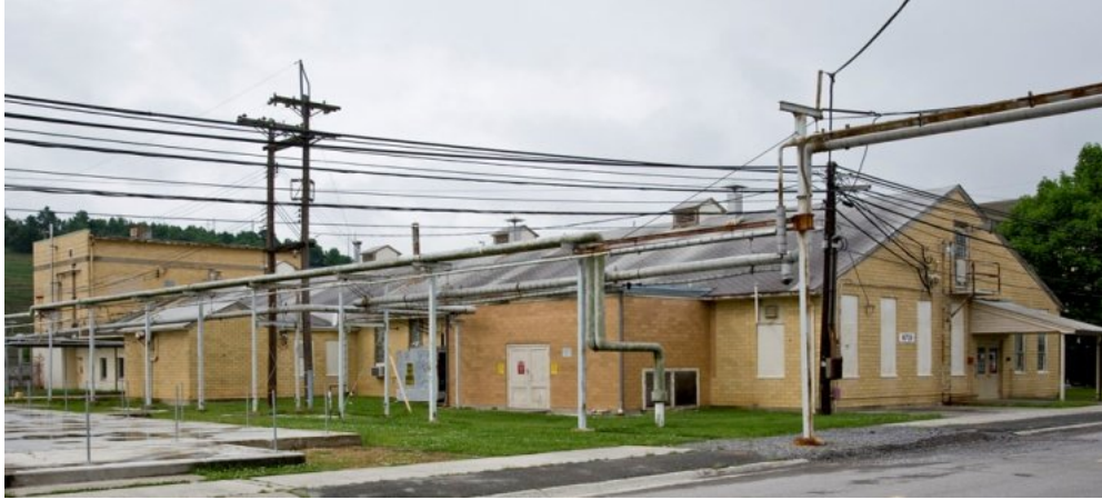
Fig. 3 Building 9735 prior to demolition by ARRA project team.
