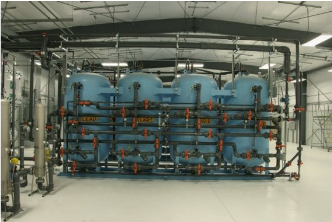
Figure 1. Modular 100gpm ion exchange “train”
