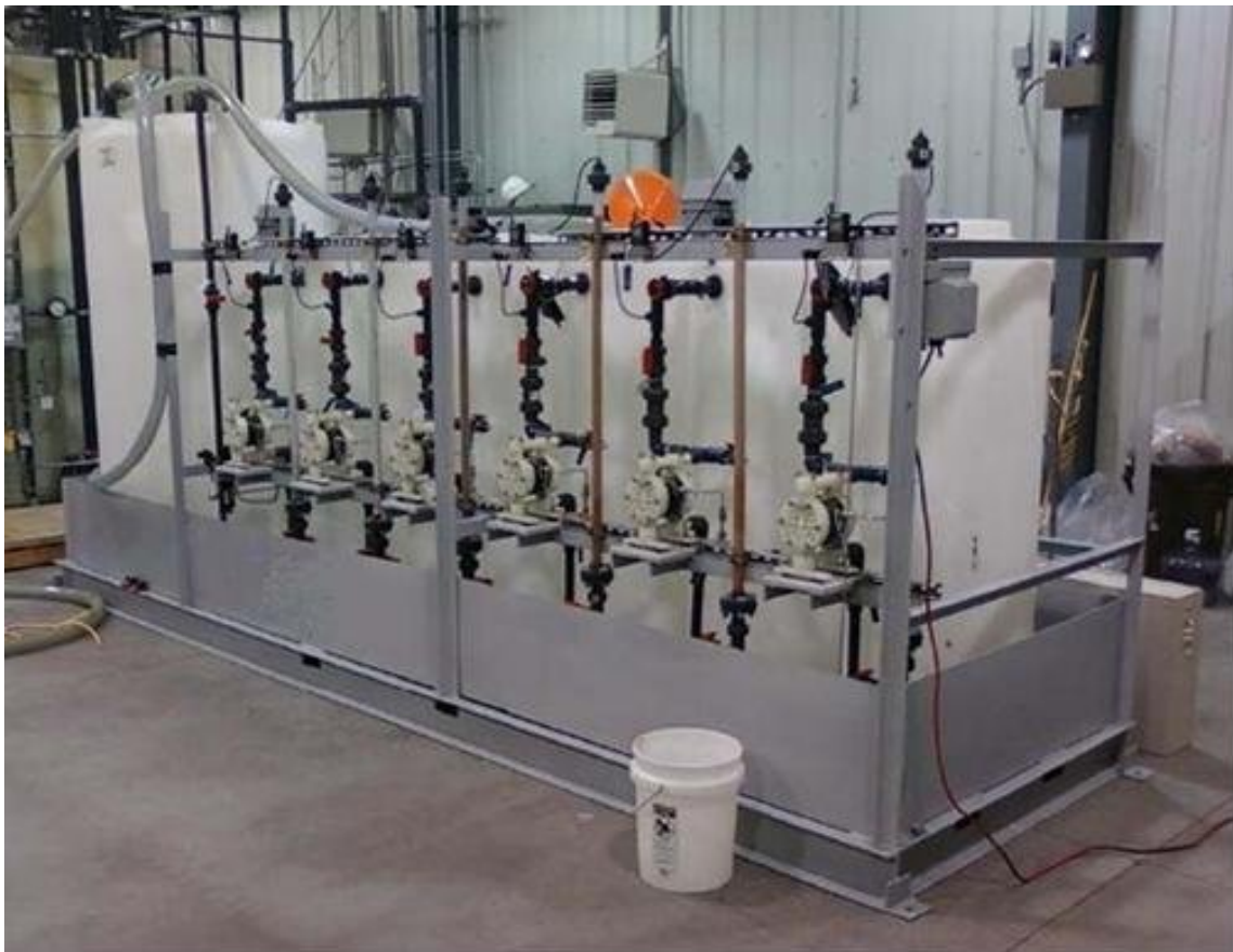
Figure 2. Resin test skid.
