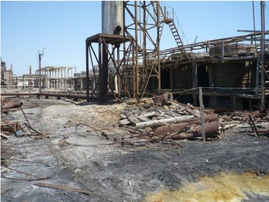
Fig.1. The shop state at the moment of the survey.
