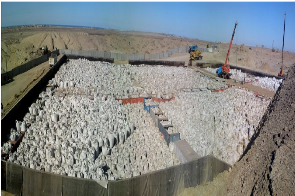
Fig. 4. Repository is filled with more than 90% of the waste.
