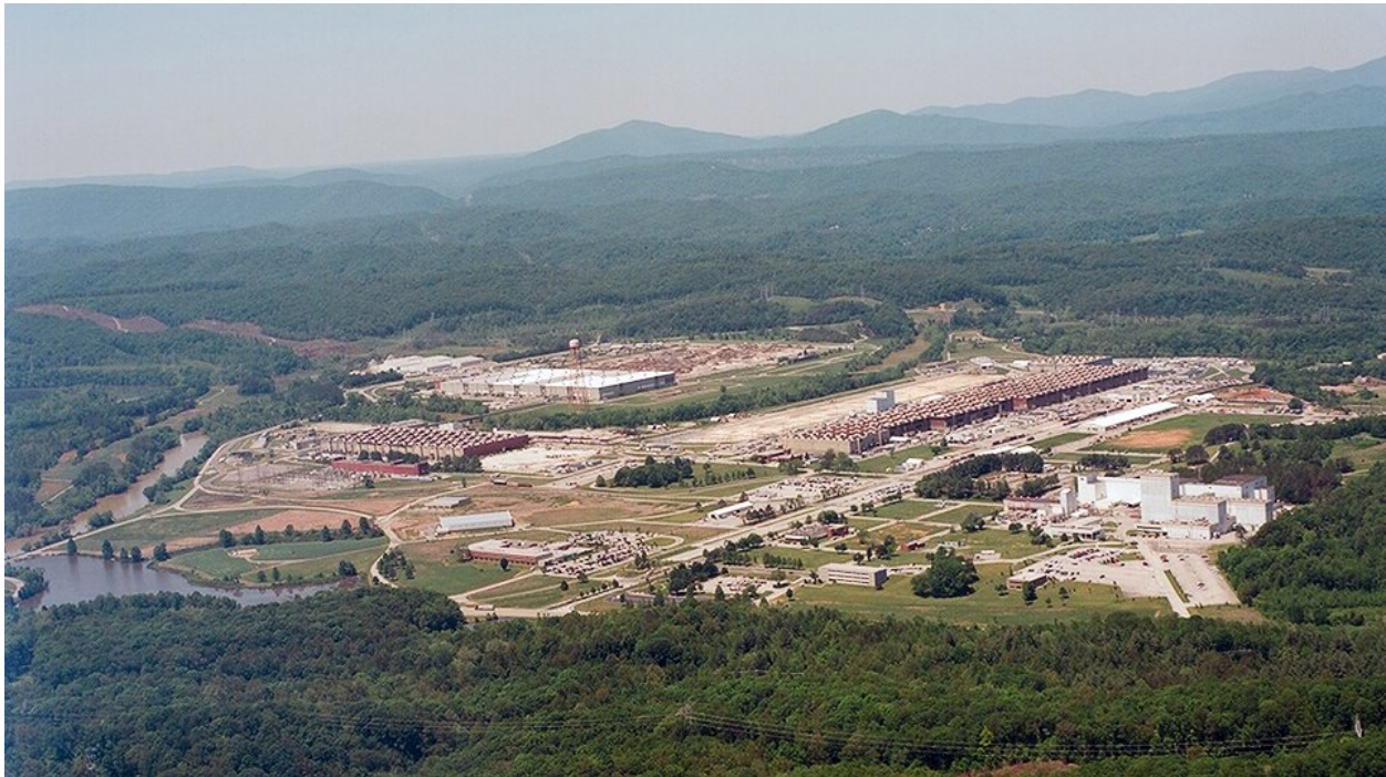
Fig. 1. East Tennessee Technology Park
