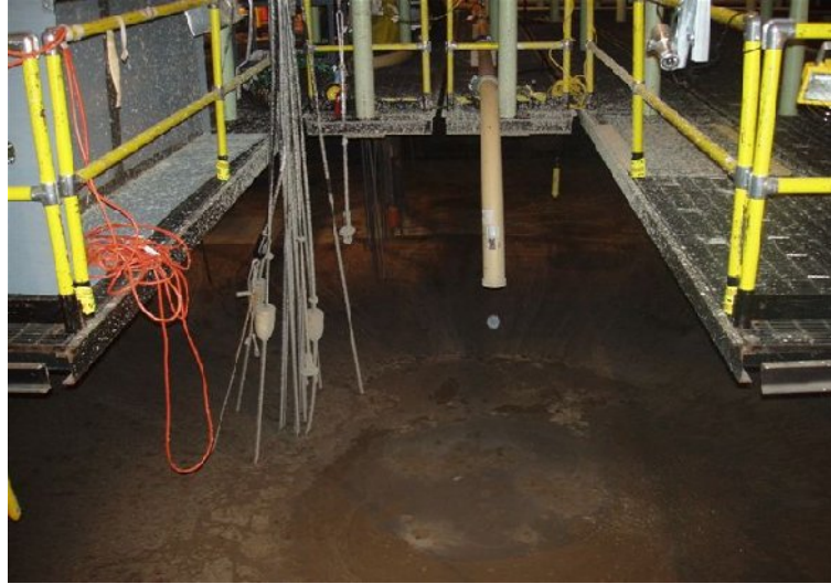
Figure 3. Remote grout placement in spent fuel storage basin through rigid piping. Personnel access was prohibited in basin throughout placement actions due to excessive dose.
