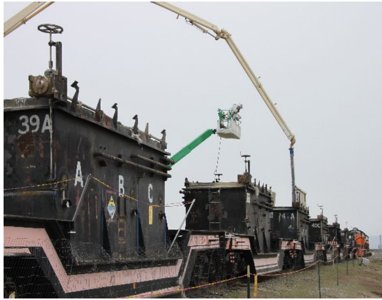
Figure 2. Grout placement into contaminated rail car vessels using remote articulated boom truck directed by personnel in aerial lift.
