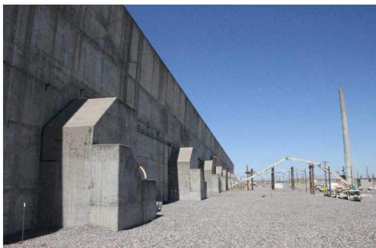
Figure 1. Articulated boom grout placement truck and transit-mix truck, off loading into chemical separations plant cells through high pressure ridged and flexible piping.
