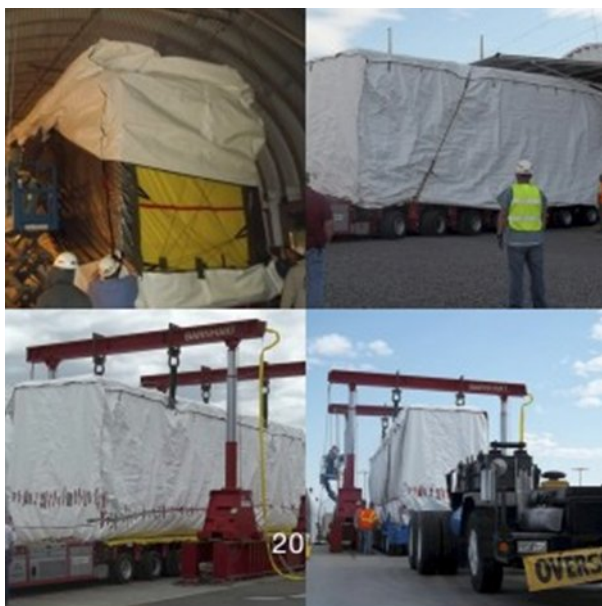
Fig. 1 Condenser Packaging, On-Site Transport and Trans-Loading in Preparation for Transport
