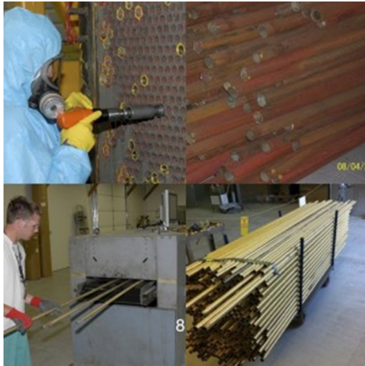
Fig.-3 Condenser Tube Disassembly and Processing
