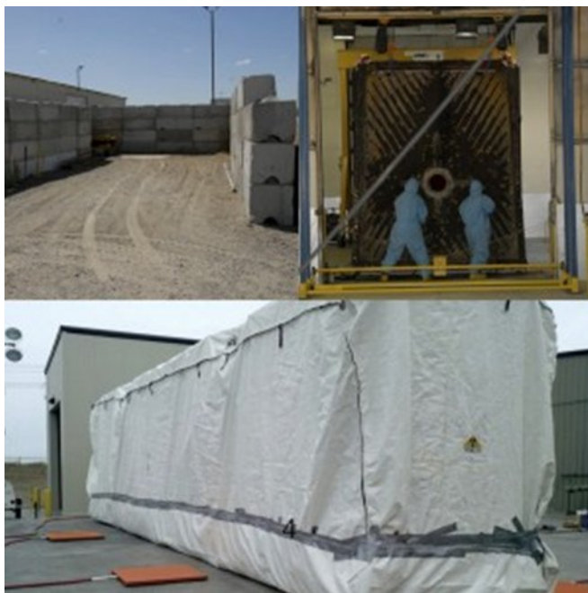
Fig.-2 Waste Processing Facility Modifications
