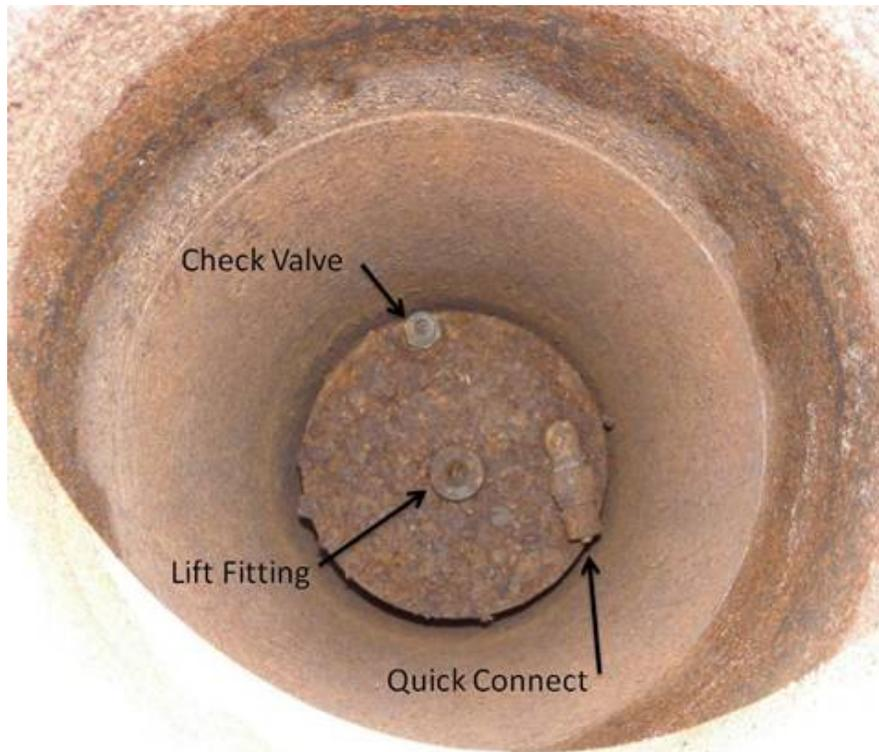
**Figure 3 Presence of Corrosion Shown on Top of a Fuel Can**
