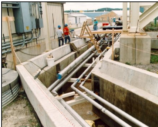
Fig IV. HLW transfer piping during installation
