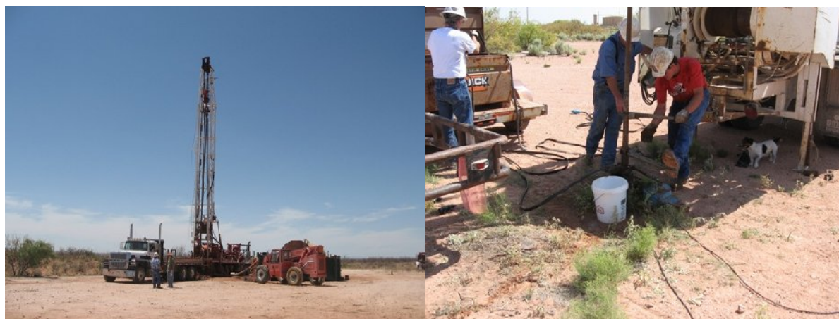
Figure 2 – WIPP Groundwater Investigations – Monitoring Well Drilling and Testing
