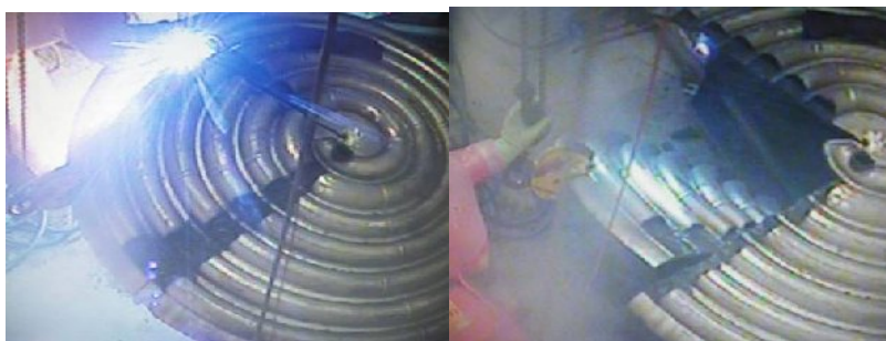
Fig. 1 Plasma torch for cutting the bottom of a dissolver from the dissolution line
