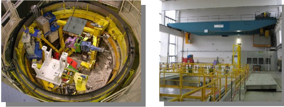
Fig. 3: The cold test rig (left) in the emptied MZFR turbine hall (right)
