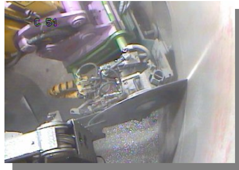
Fig. 7: Segmenting of the liner by means of the universal cutter
