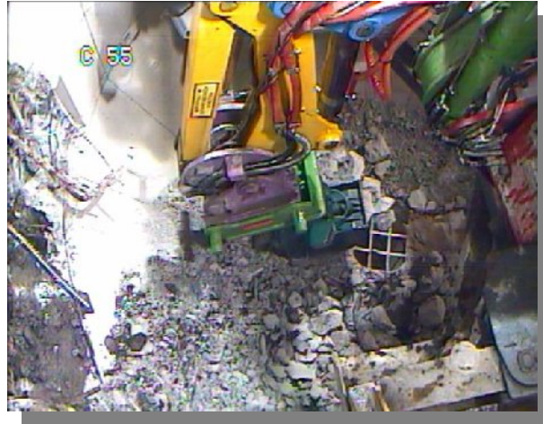
Fig. 10: Transfer of the concrete rubble to the packaging station via the vertical borehole
