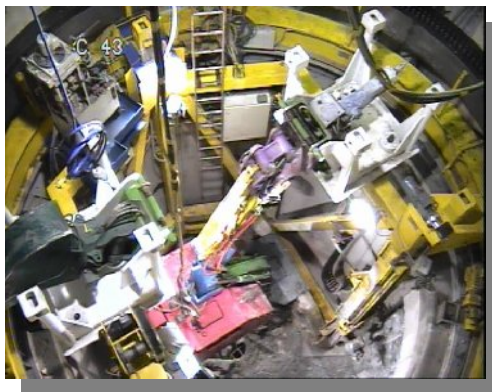
Fig. 8: Excavator in working platform during tool transfer
