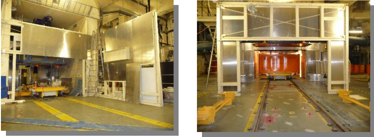
Fig. 4 Installation (left) of the packaging facilities for activated concrete on level +0 m. The right figure shows the complete installation of the packaging facilities with open gates and a container in the background from the perspective of the material lock
