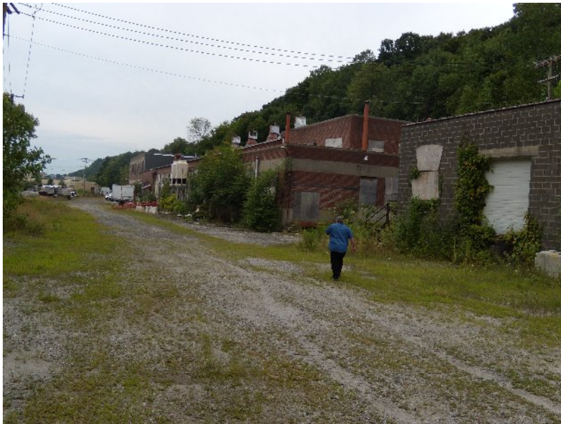
Figure 8. DOE inspects the Seymour, Connecticut, Site where supplemental limits were imposed.
