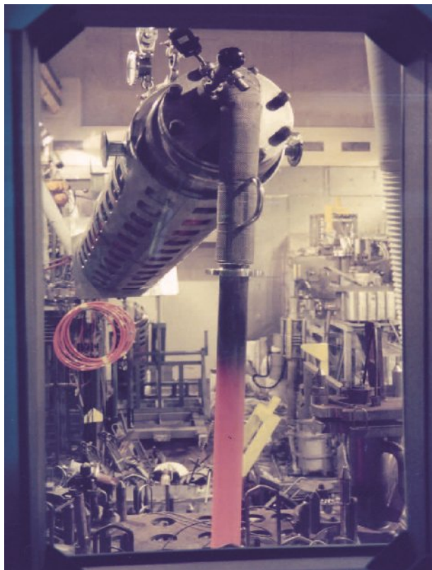
Fig 3. Evacuated canister removing molten glass from melter cavity
