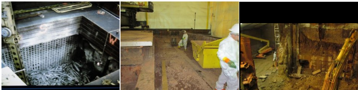
Figure 2 - Brookhaven (Full remote core removal, semi-remote roof removal, fully manual bio-shield removal)
