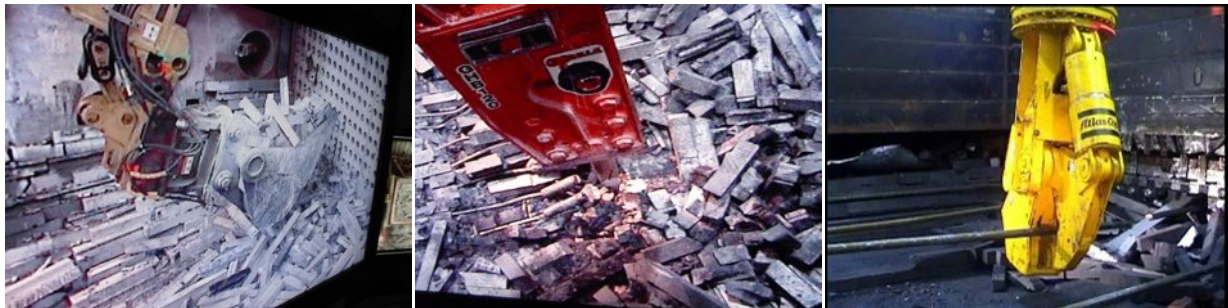
Figure 3 - Core removal using bucket, hammer and shear
