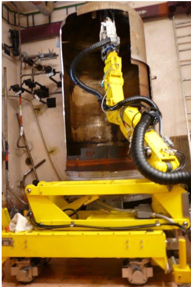
Fig. 4. Dismantling of the evaporator by MT80A manipulator.
