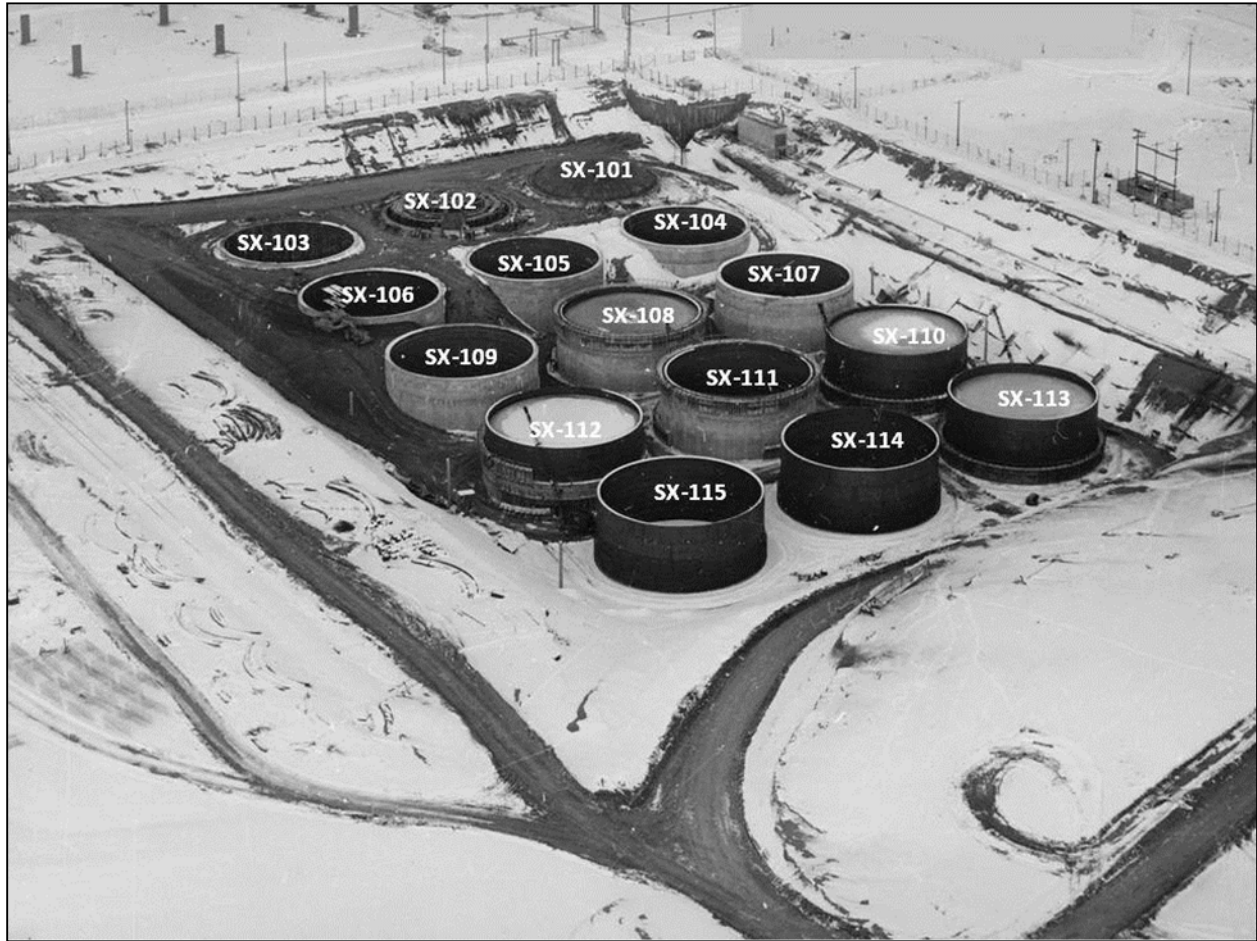
Figure 5. SX Farm Construction Photograph January 20, 1954 (N1D00585052)
