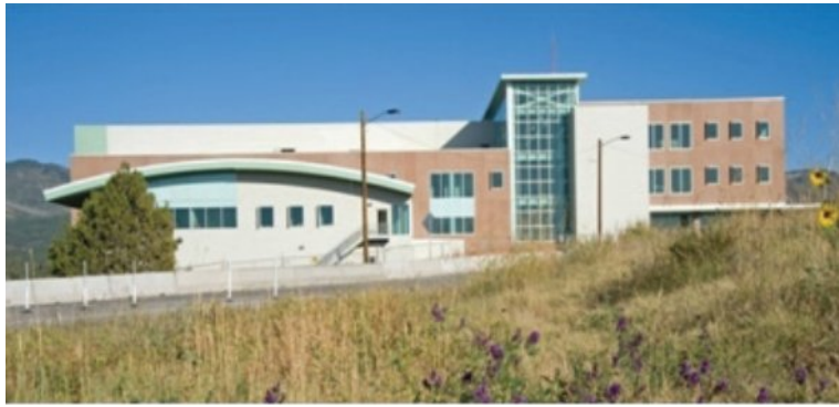
Fig. 3. Radiological Laboratory/Utility/Office Building (RLUOB)
