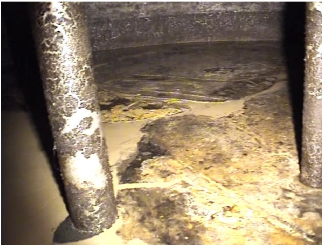
Figure 1: Internal view of resin vault
