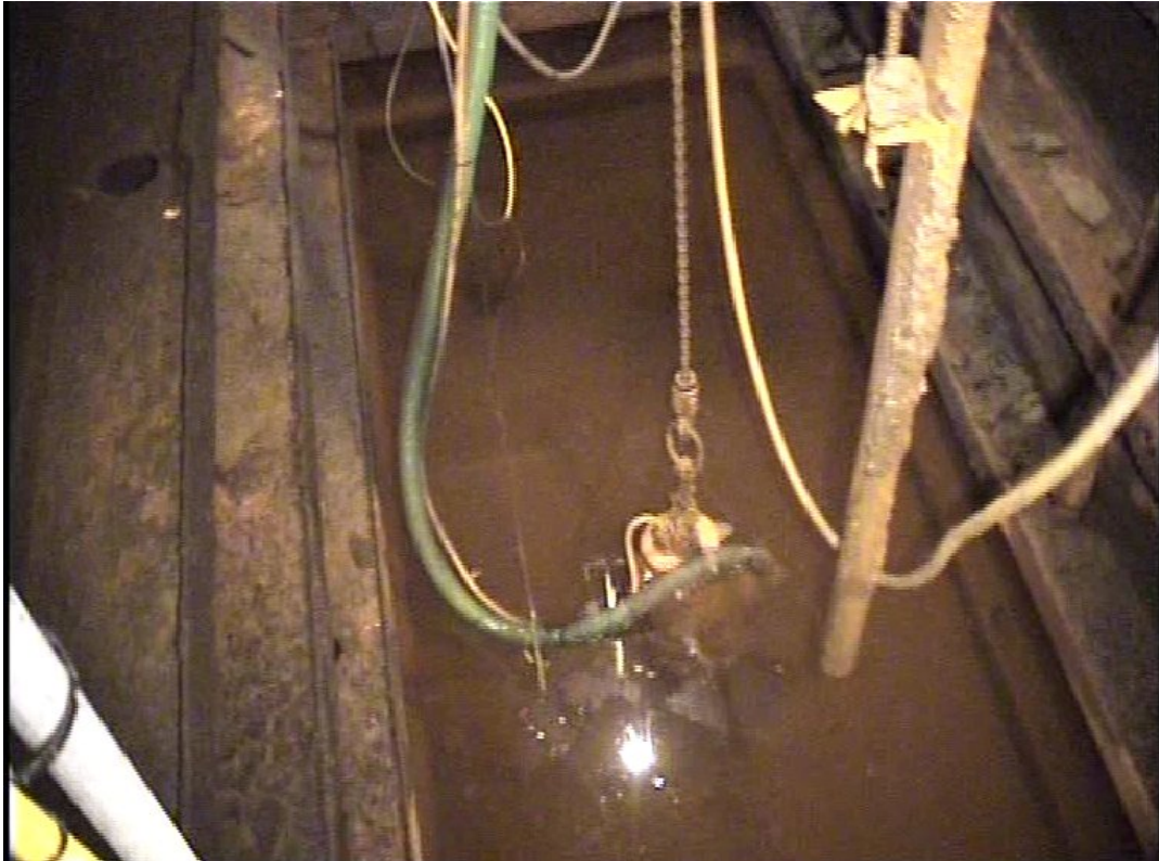
Figure 2: Internal view of main sludge vault
