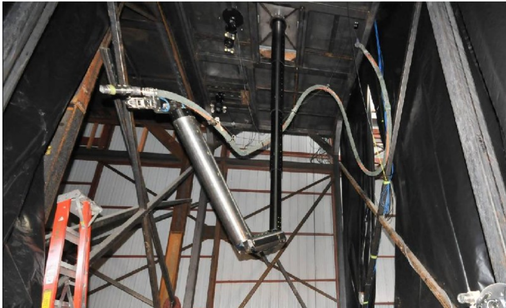
Figure 3: RDA during testing of bulk hose management
