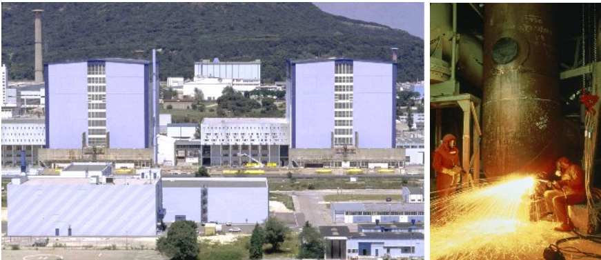
Fig. 3 and 4: view of G2 and G3 reactors in 2009 (left) and dismantling operations (right)
