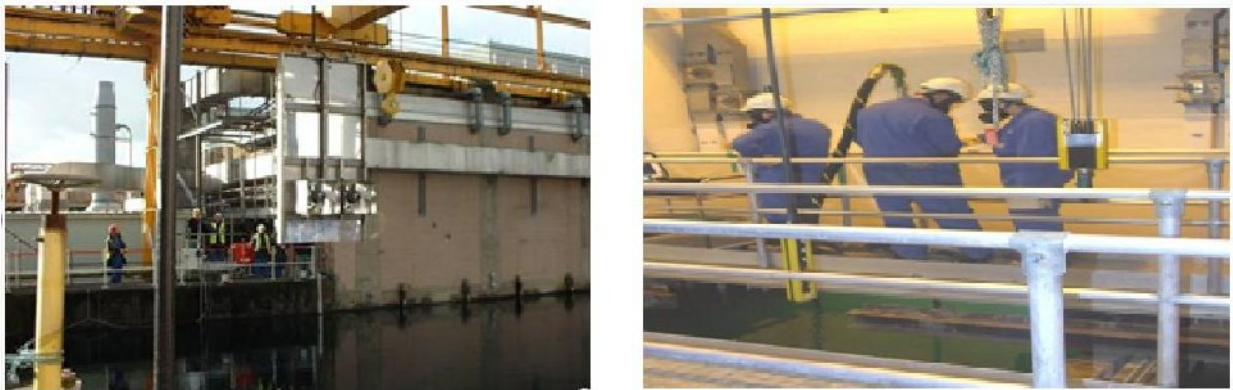
Figure. 2 Bay desludging operations
