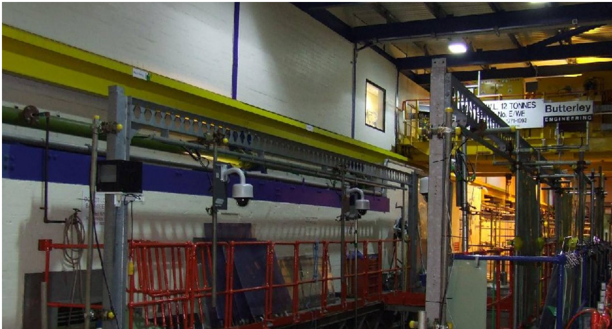
Figure 5. Plant ready for transfer
